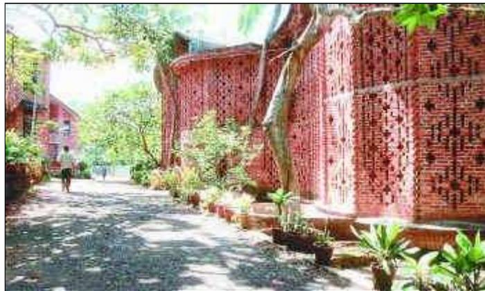
**The Computer centre at the Centre for Development Studies, Thiruvananthapuram. Here Baker evolved an innovative system of curved double walls to save on cost and to conserve the energy that goes into air-conditioning a building of this scale and purpose.**
